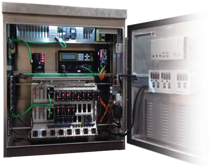
Sturdy .125" 5052-H32 aluminum cabinet with three-point Number 2 APL lock standard.
