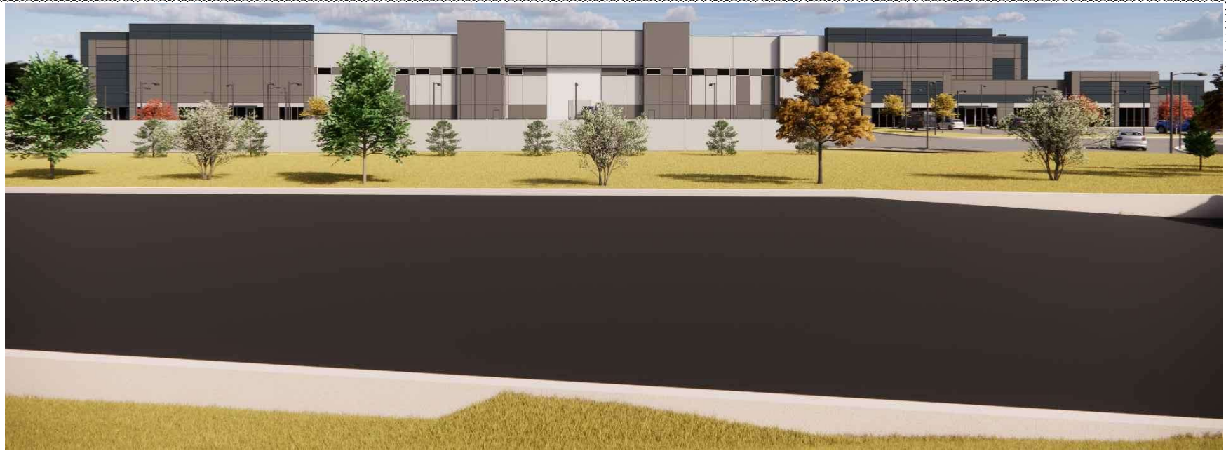
⑥ FTI - MECHANICAL 2 - SOUTH VIEW
