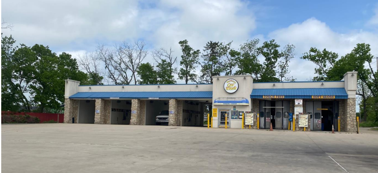
View of the subject property looking north.
