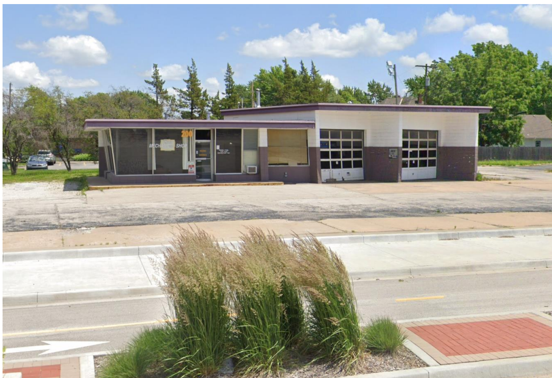
View of the Property Looking East from S. Kansas Avenue
