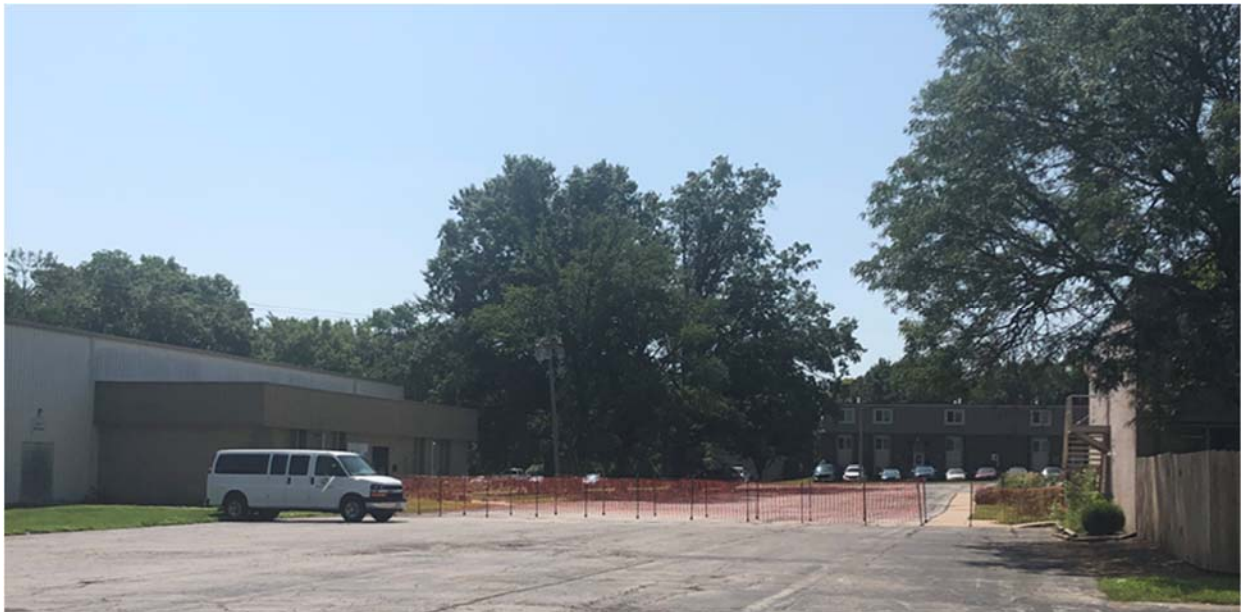
(View of proposed building addition space from north parking lot.)
