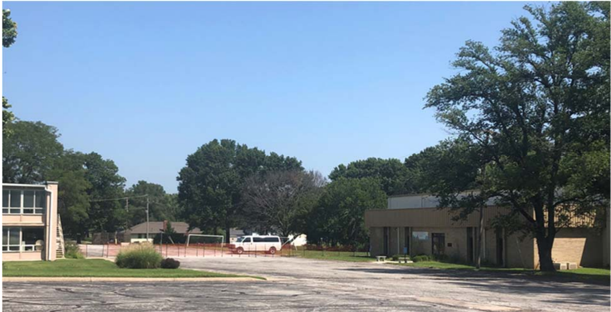
(View of proposed building addition space from south parking lot.)
