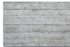
Board Form Concrete
