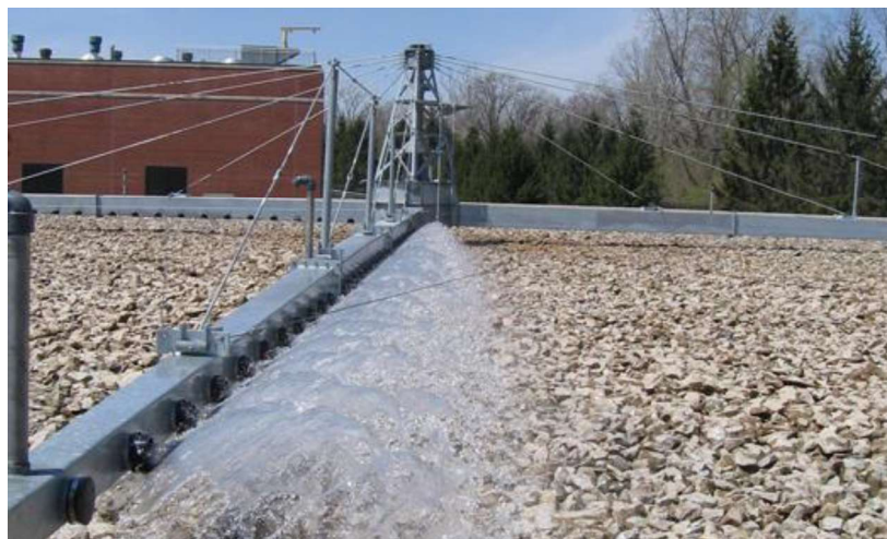
A 200-foot diameter WesTech Rotary Distributor unit designed for up to 17,500 gpm.
