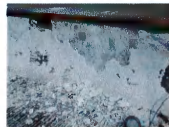
Hollow, deteriorated pool plaster removed Kansas City, KS
