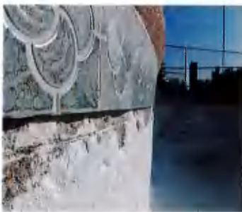
Saw-cut and chip below tile
