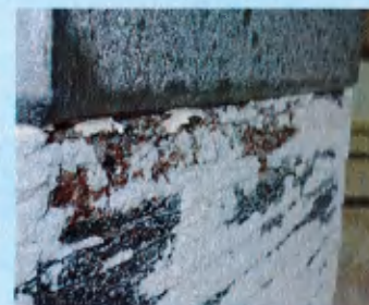
Removal of soft and deteriorated plaster at Prairie Band Potawatomie Indian Nation, KS
