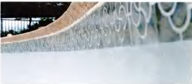
New plaster flush with tile. No ugly bulge.
