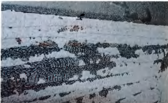
Pool Surface After Hydro-Blasting
