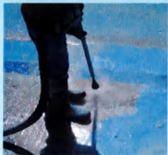
Hydro-Blasting in Action
