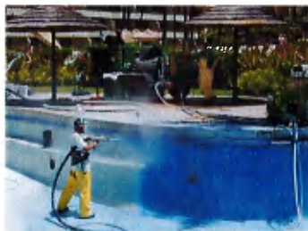
Hydro-Blasting removing pool paint
