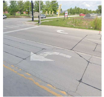
▲ Induction Loop Detectors
