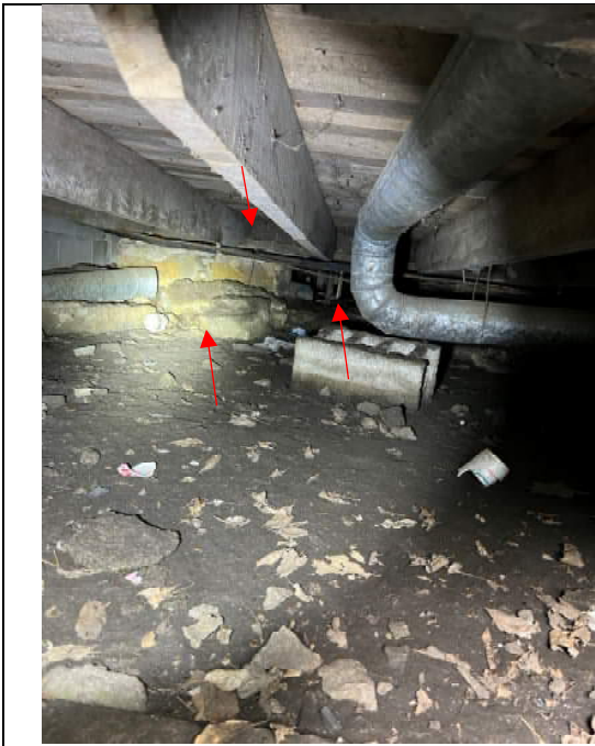
Photo 9: Southeast wing framing. Note the flush beam, stone remnants, and jack post
