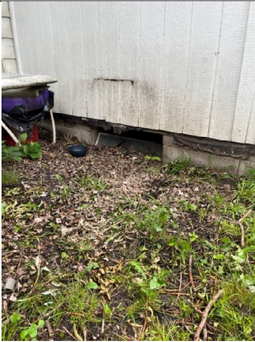
Photo 5: Crawl space access
