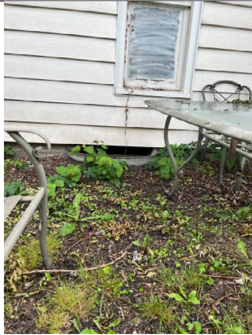
Photo 6: Crawl space access
