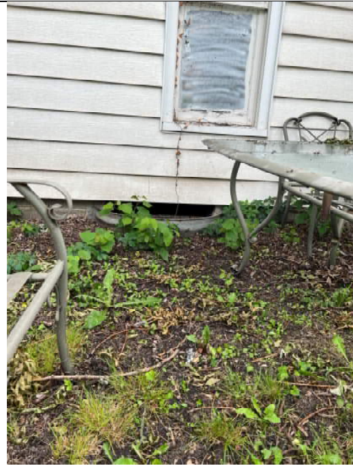
Photo 6: Crawl space access
