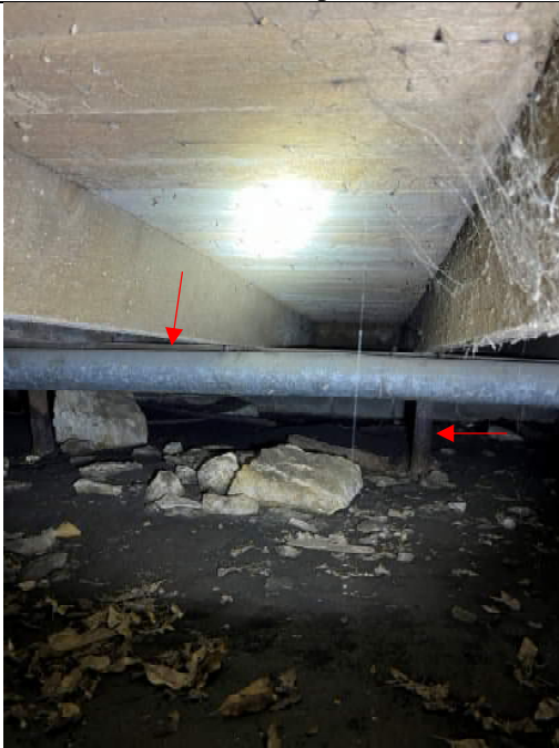
Photo 7: Northeast wing framing. Note the beam and short post
