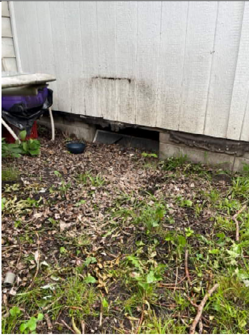
Photo 5: Crawl space access
