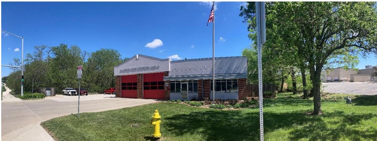
View of the subject property looking northeast from Mur-Len Road.
