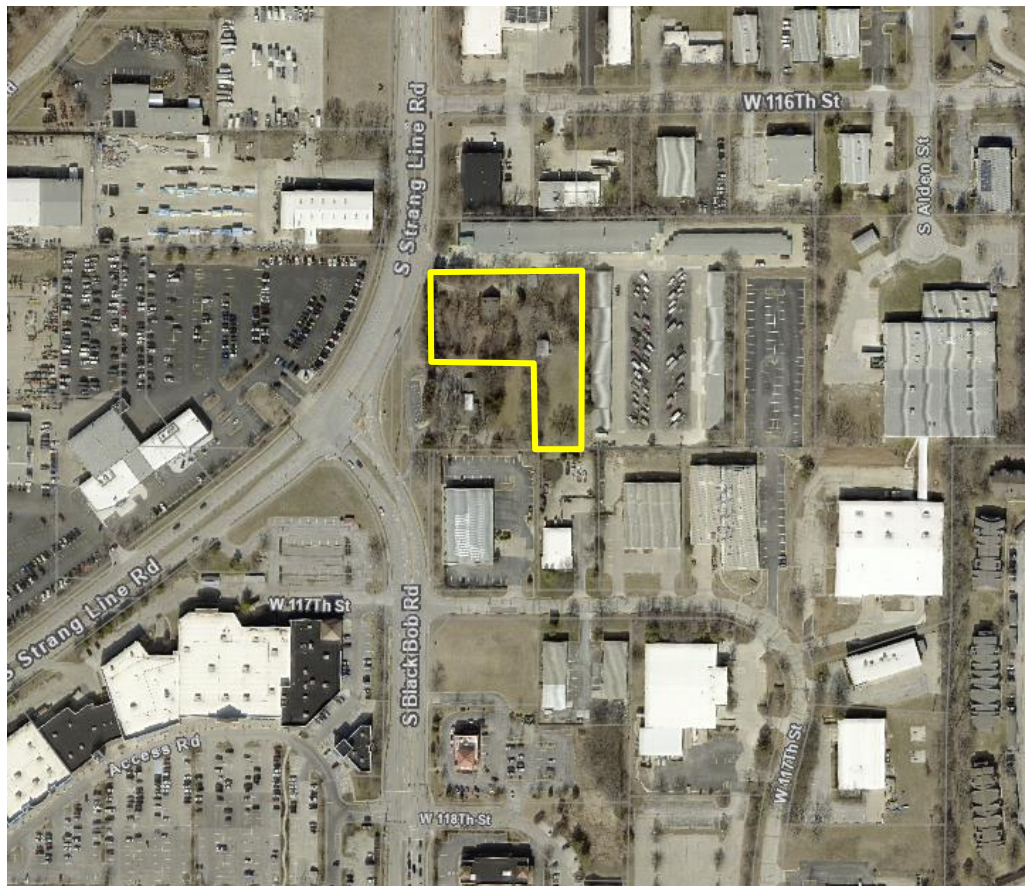
Aerial view of the subject property highlighted in yellow.
