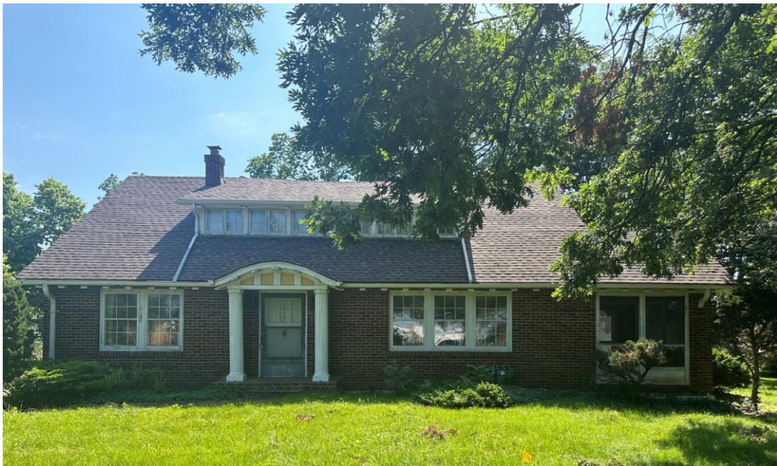
Primary Façade – west elevation.
