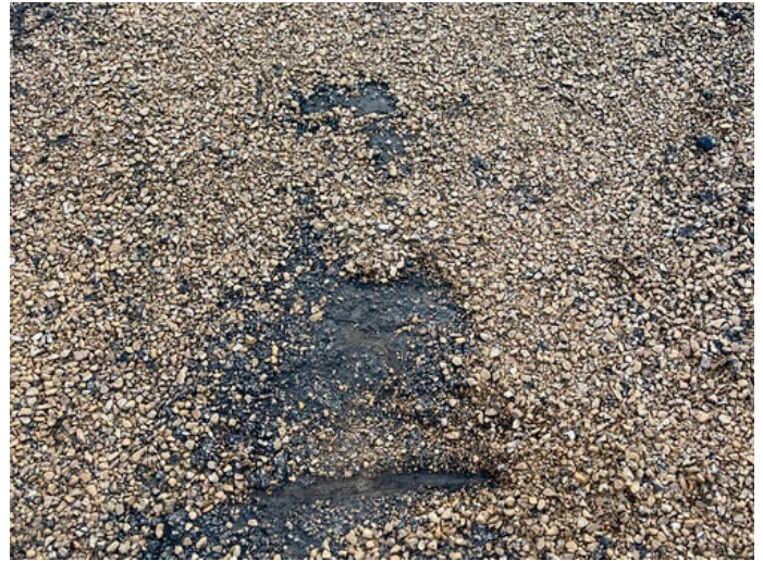
Cracks in membrane
