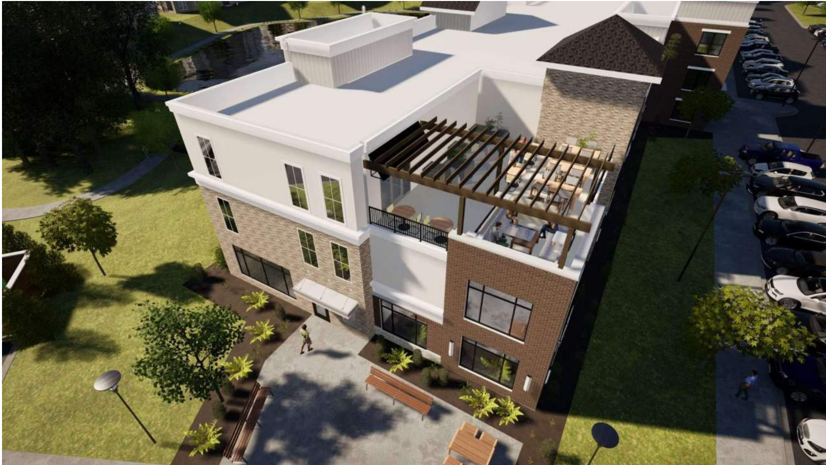
VIEW AT ROOF TOP / PLAZA AT BUILDING 2
