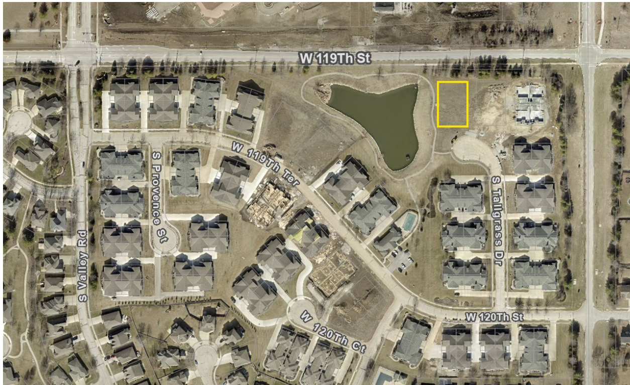
Aerial View of the Subject Property (Yellow)
