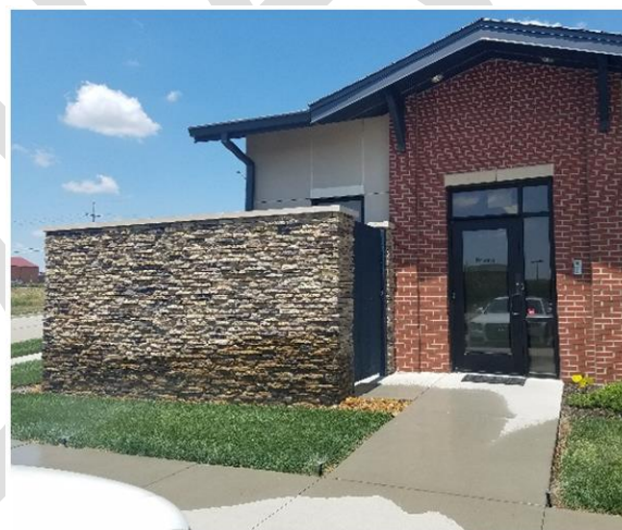
Decorative Wall Screening at Building
