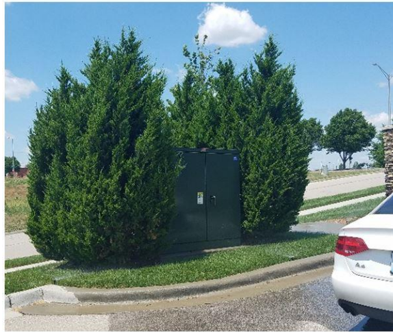
Adequate Three-Sided Screening
