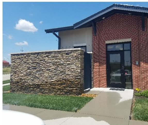
Decorative Wall Screening at Building
