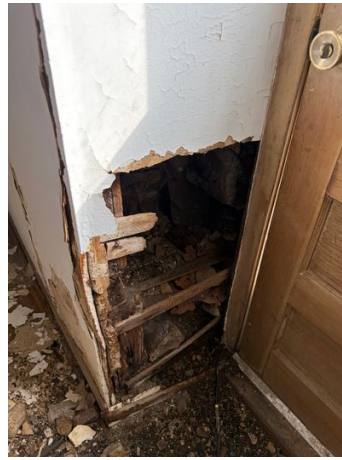
Image: 8: Deterioration at the northeast corner of the roof
