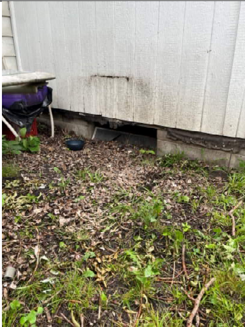
Photo 5: Crawl space access
