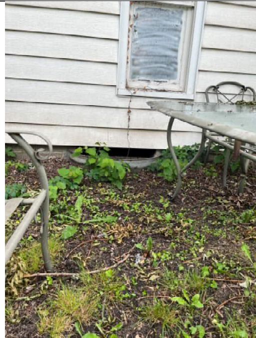
Photo 6: Crawl space access
