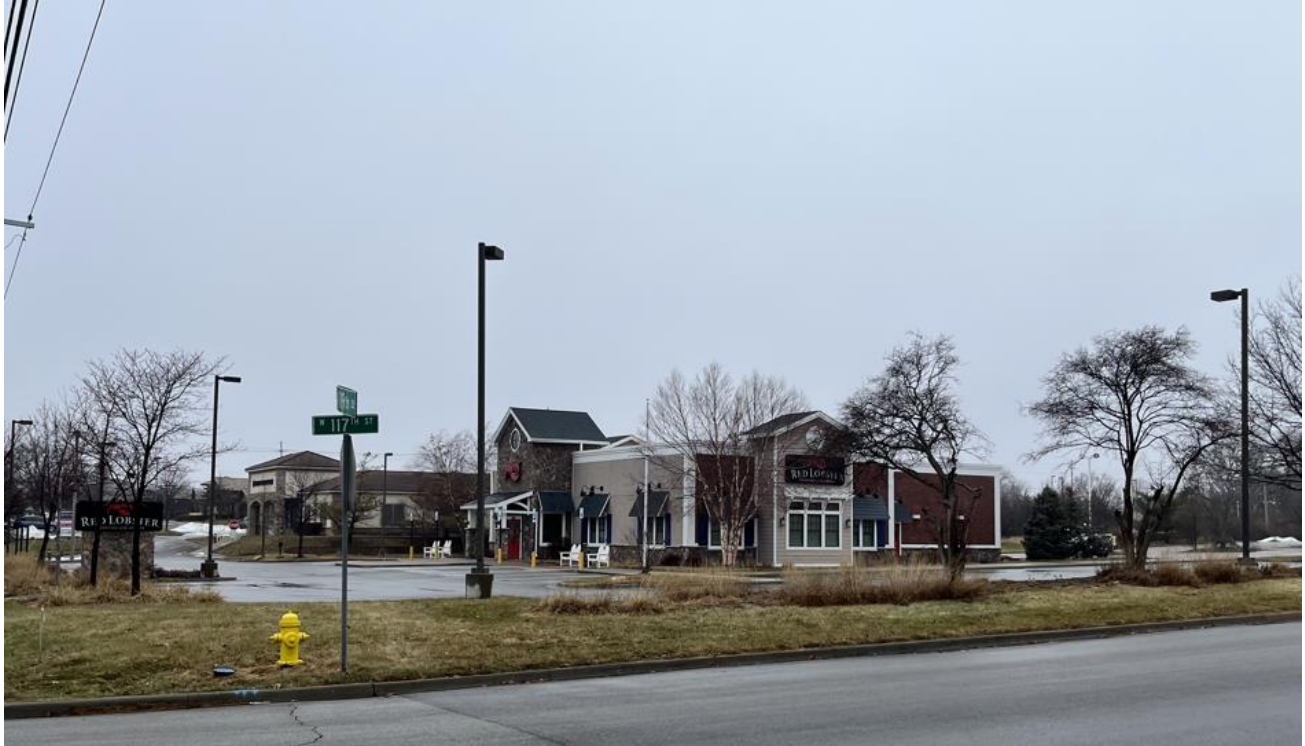
View of subject property looking northwest.
