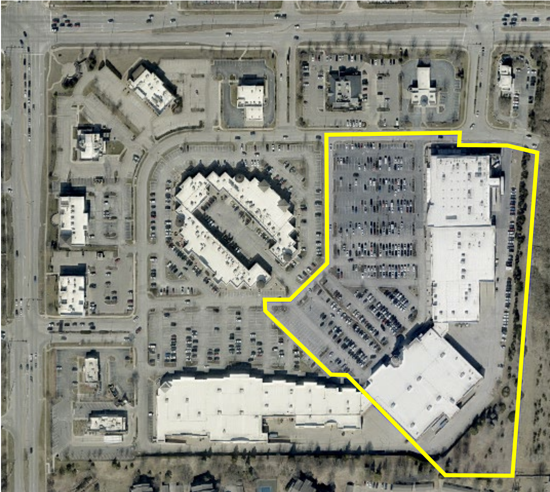
Aerial view of the subject property outlined in yellow.
