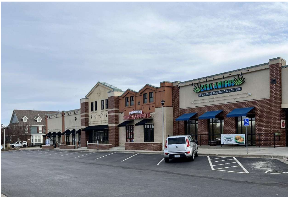
View of subject property looking southeast.
