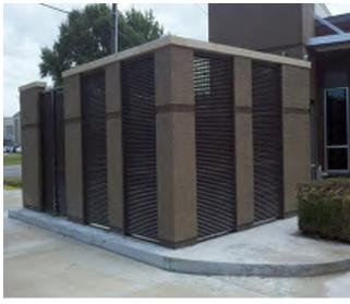
Architectural screenwall utilizes mixture of materials and is complimentary to adjacent architecture.
