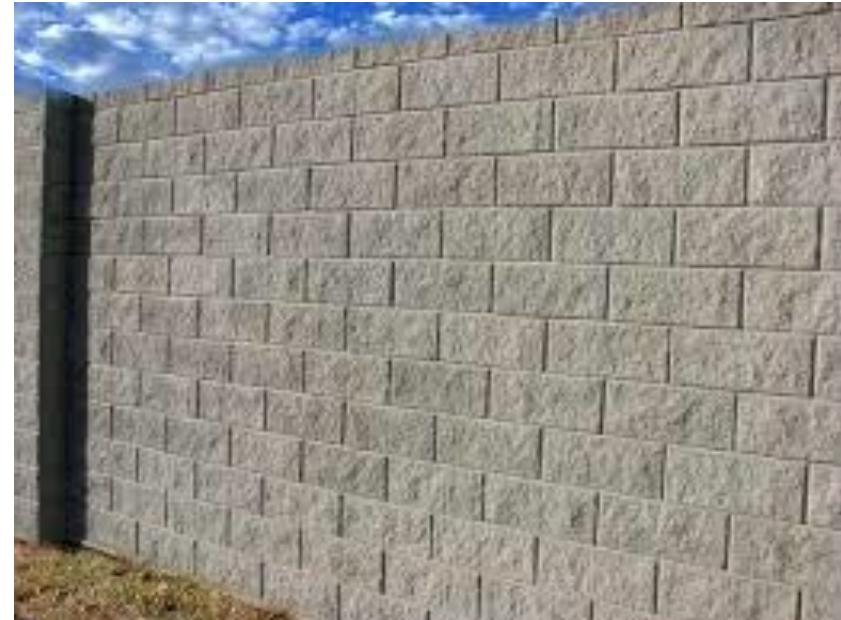
SPLIT FACED CMU MASONRY
