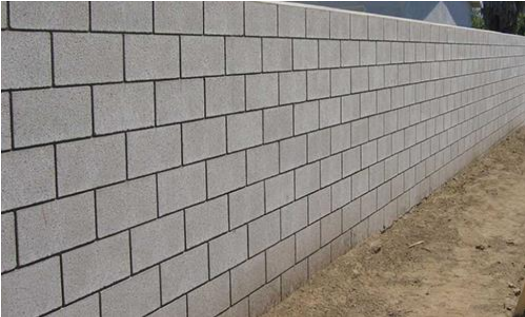
BURNISHED BLOCK MASONRY
