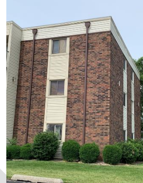
Examples of exposed downspouts on primary façade
