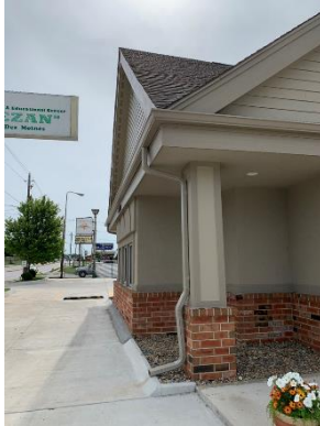
Example of exposed gutter and downspout on primary façade
