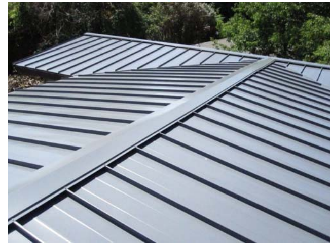
STANDING SEAM METAL ROOF
