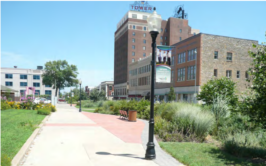
Downtown bioswale in Topeka. This innovative project replaced an unnecessary travel lane.
