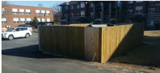
Vertical wood slat fencing is prohibited as a screening material and shall not be utilized in the Mentum Development.
