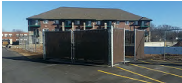
Chainlink fencing is prohibited as a screening material and shall not be utilized in the Mentum Development.
