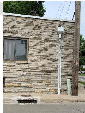
Examples of exposed downspouts on primary façade
