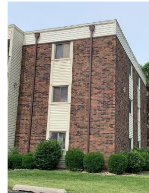
Examples of exposed downspouts on primary façade
