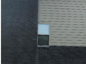
Example of window missing trim on one side
