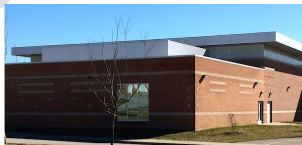
Roof top mechanical equipment appropriately screened
