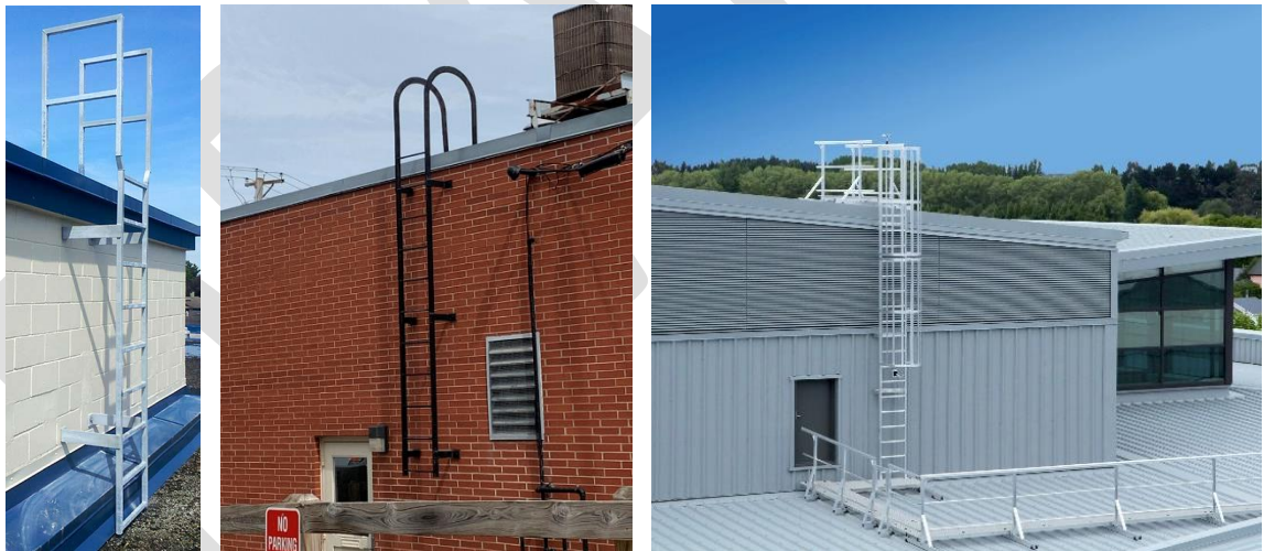
Examples of exposed exterior roof access ladder
